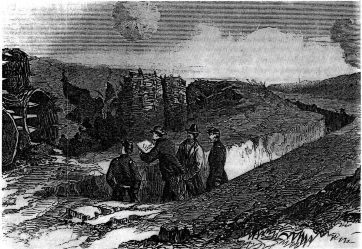
Fred. B. Schell shows himself in the trenches before Vicksburg sketching the mining operation of Fort Hill. According to the text accompanying this engraving, "the sketch was made in the sap within 15 feet of the rebel Fort Hill, behind which lay the rebel sharpshooters, held at bay by Coonskin and other riflemen, eagerly on the look-out for a rebel head" ( Leslie's , July 25, 1863, pp. 273, 290).
